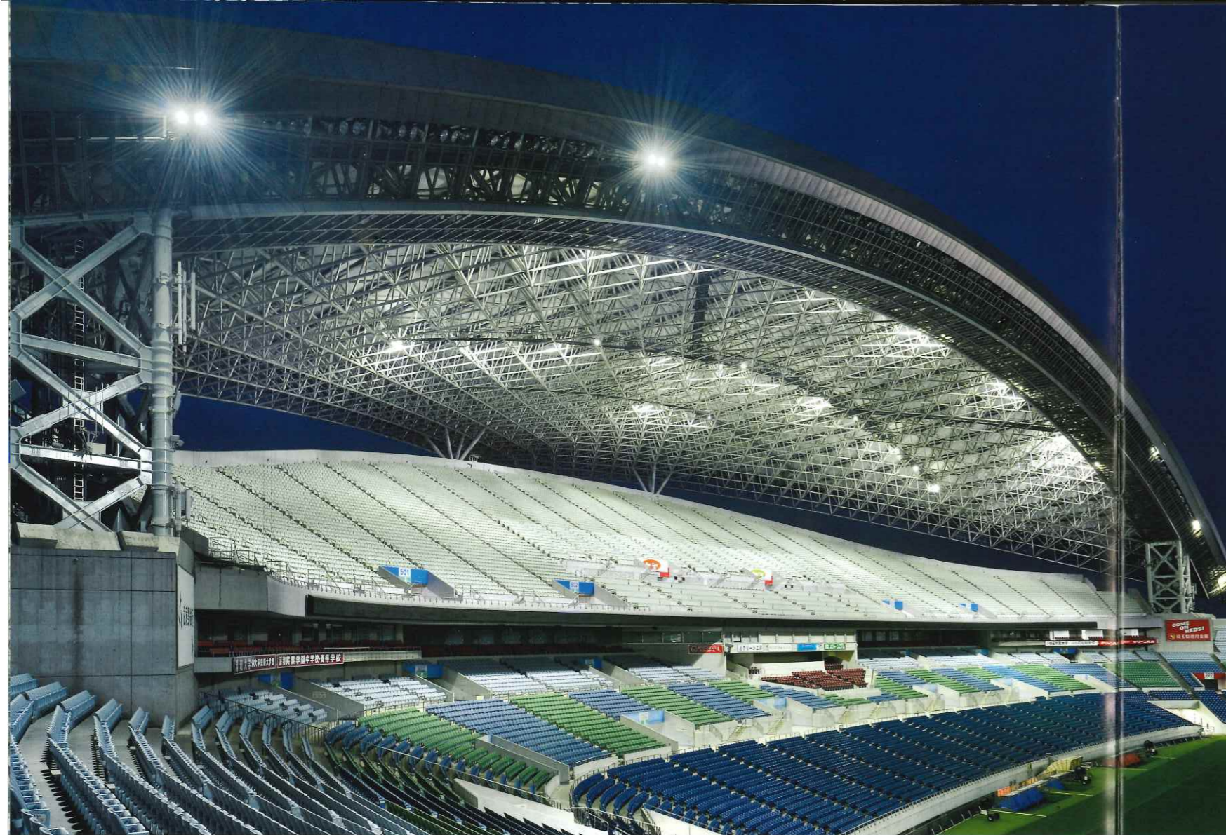
2羽の白鷺(しらさぎ)をイメージした膜屋根が特徴的なスタジアムのメインスタンド側をのぞむ。 A view of the main-stand side of the stadium, which is characterized by a membrane roof in the image of two white herons.
